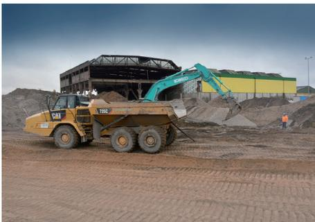
The overall project has an investment volume of about € 7.8 million. Construction activities include the demolition of about 13,000 m<sup>2</sup> of hall space, civil engineering and road works, drainage, lighting and security measures for the area. The application of a new asphalt coating which is currently in progress will result in certain sections being ready for operation as of this April already.
